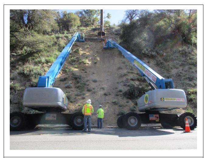
**Photo 6:** A crew installing fiber rolls and preparing to apply hydro-mulch on the steep slope at Z118138 (TL6957) to prevent erosion, in accordance with the Erosion Control Plan and SWPPP.
