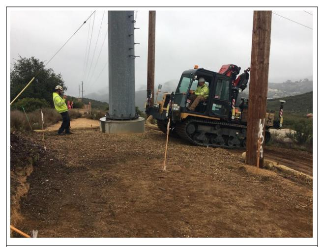
**Photo 1**: Crews position a crane atop pole site Z105008 (TL6957) in order to set up a drilling platform and associated equipment to drill micropile foundations. Biologists were observed on site working with crews as they set up within the work limits, in accordance with MM BIO-1 and MM BIO-22. Straw wattles moved for equipment mobilization were observed reinstalled in accordance with the SWPPP (MM HYD-1).
